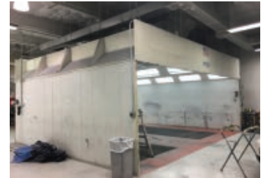
Prior to installing one of the custom double prep stations at Lexus of Pembroke Pines .
