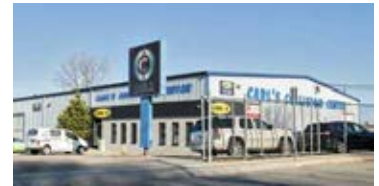
Carl's Collision repairs approximately 150 cars weekly out of two buildings totaling 40,000 sq. ft.
