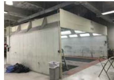
Prior to installing one of the custom double prep stations at Lexus of Pembroke Pines .
